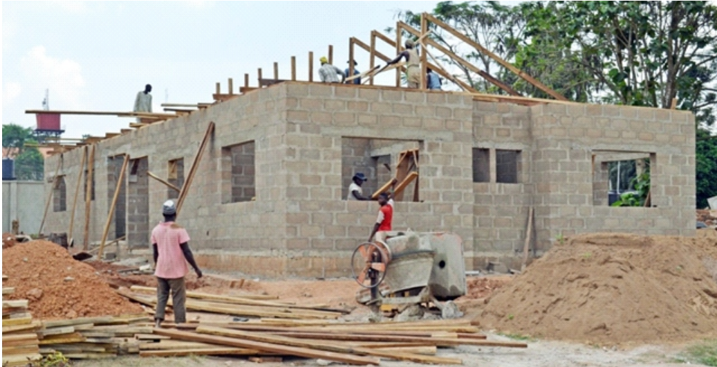
Plate 5. Residential Quarters for Tow Female Hostel Supervisors, as at Thursday, 4 December 2014
